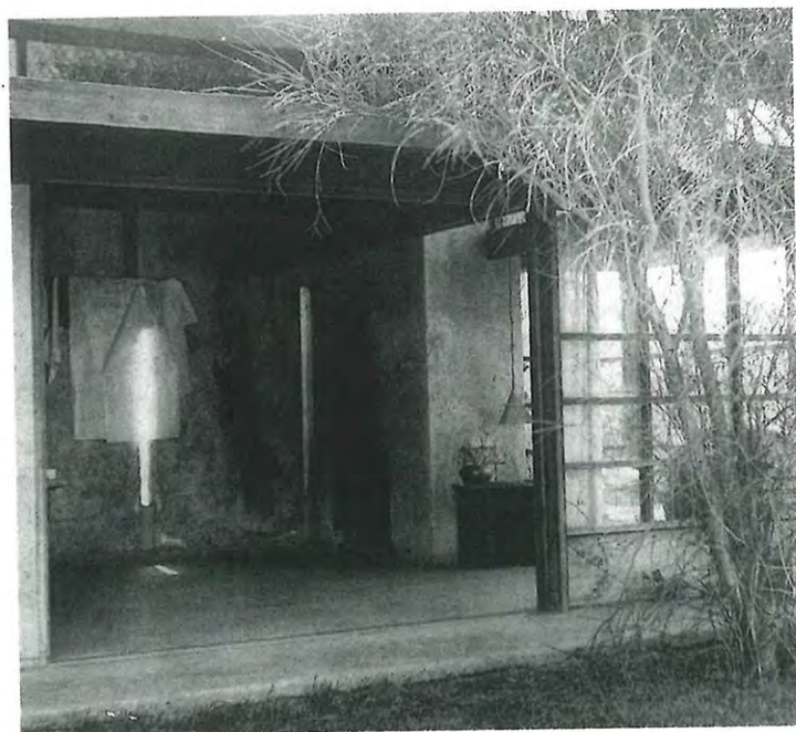
R. M. Schindler studio, ca. 1925–27. Note the use of the concrete pad as the studio floor and its extension into the court, linking interior and exterior space
