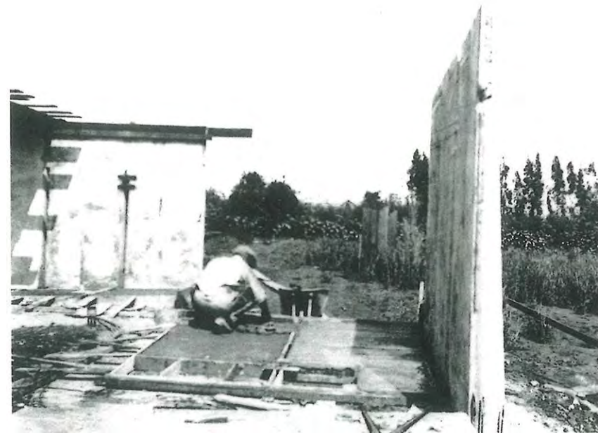
Forming a concrete slab on the concrete pad, ca. March 15–30, 1922
