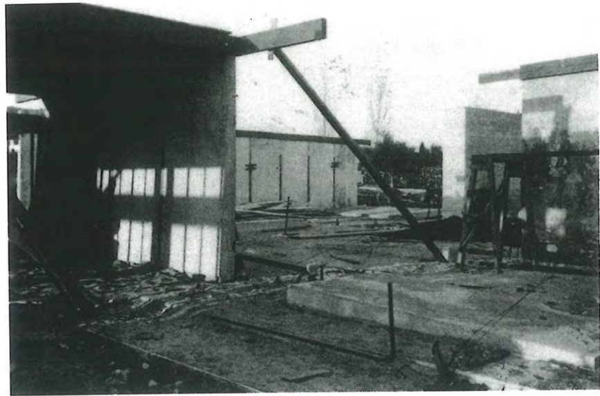
Wall and roof construction, ca. April 6-24, 1922
