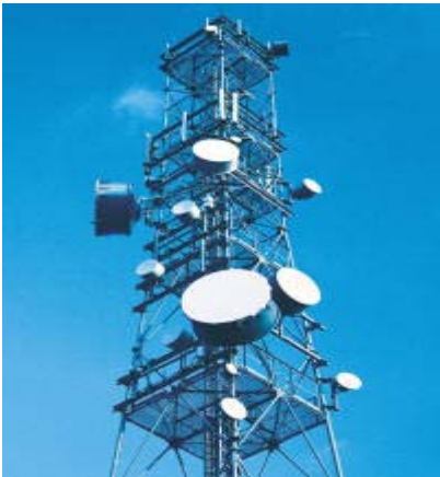
Figure 6.4 : Terrestrial Microwave:
