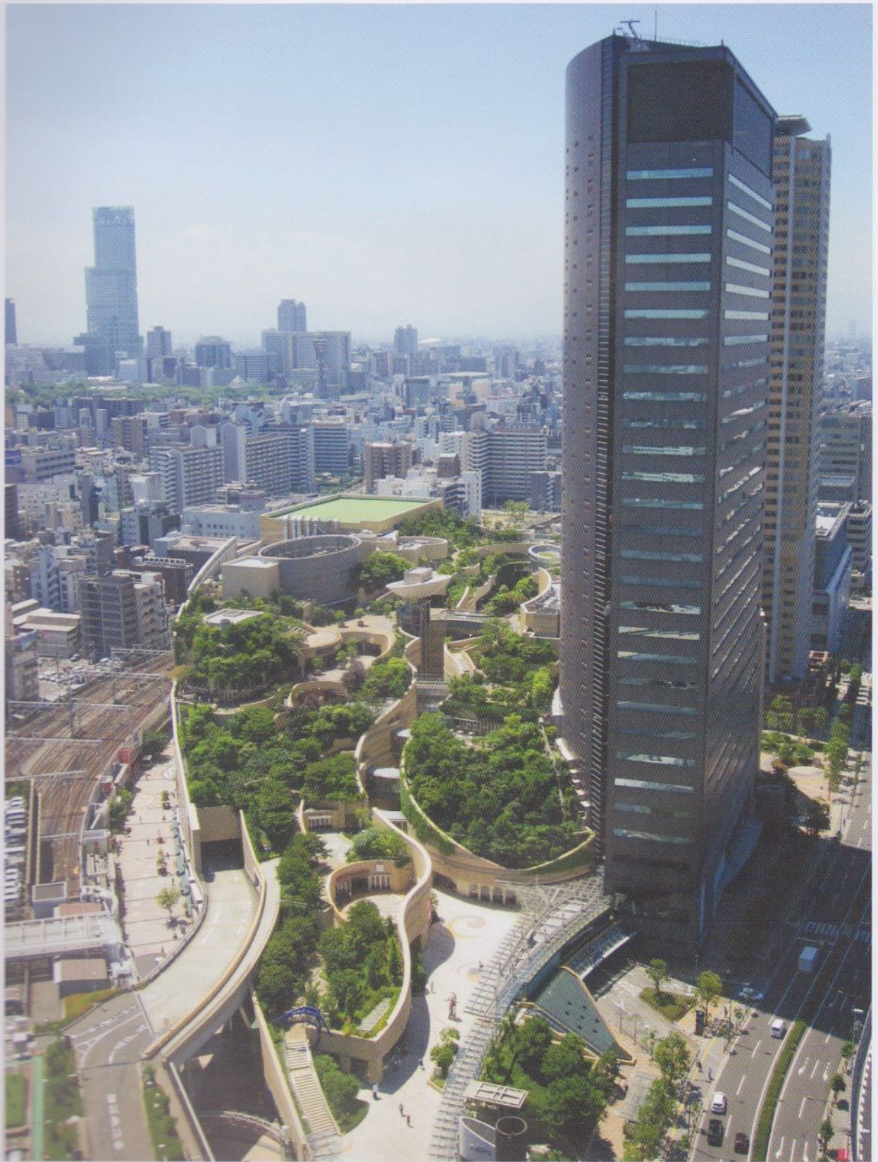
1.15 Large-scale terraced roof-top park—Namba Parks, Osaka, Japan.
