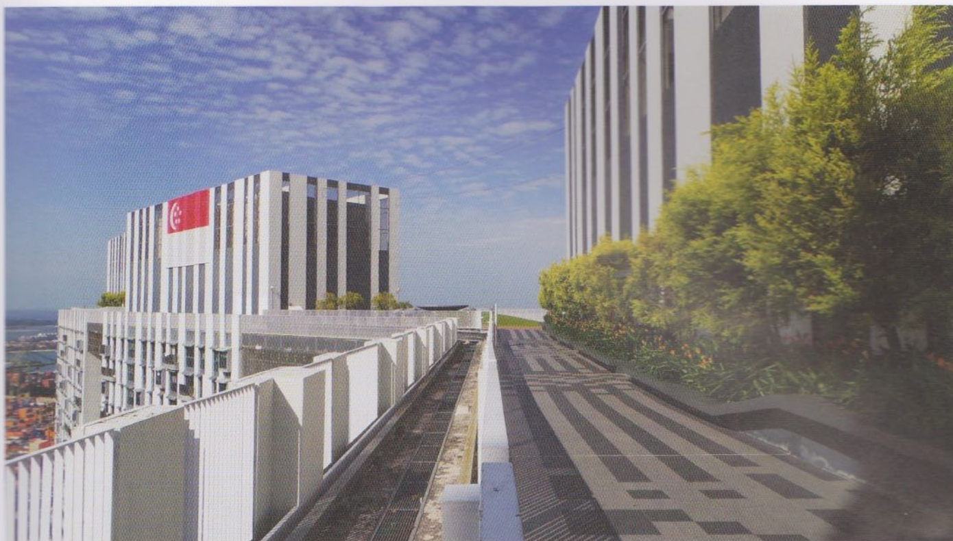
1.1 Elevated public space (sky bridge)—Pinnacle@Duxton, Singapore.
