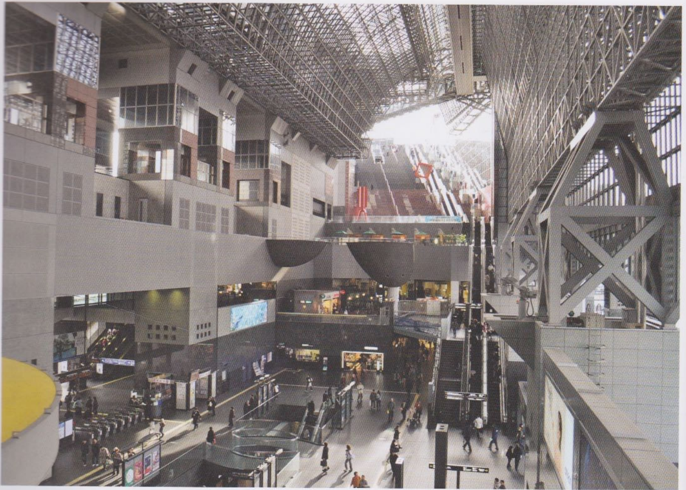
1.10 Multi-functional transit hub—Kyoto Station, Osaka, Japan.
