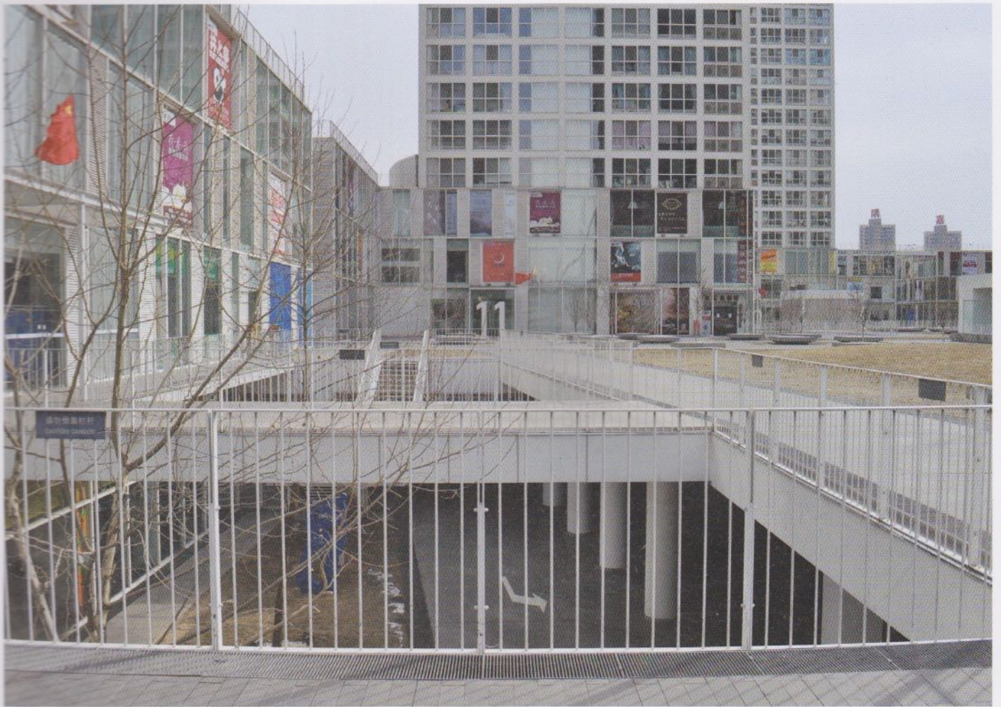
1.2 Multi-level network of public spaces—Jianwai SOHO, Beijing, China.
