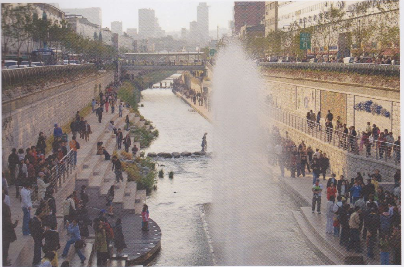
1.19 Sunken parkway—Cheonggyecheon stream, Seoul, South Korea.
