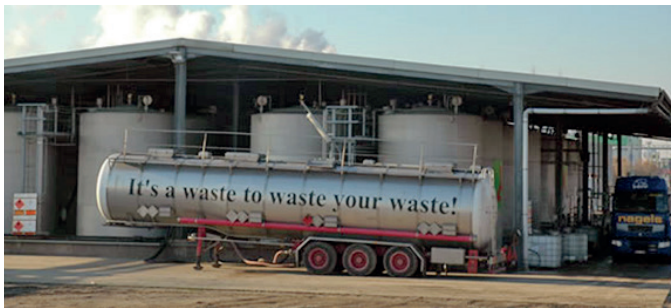
Fig. 3. Courtesy of De Neef Chemical Processing, Belgium
