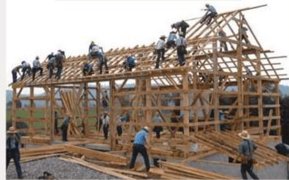
An Amish barn raising in Tollesboro, Kentucky.
